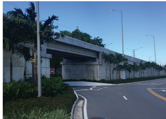
Fig. 1 Constructed MSE Walls
