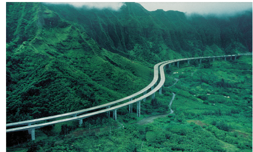
Interstate H-3, Oahu, Hawaii: ASCE recognized this Sierra System project with the Outstanding Civil Engineering Achievement Award.
