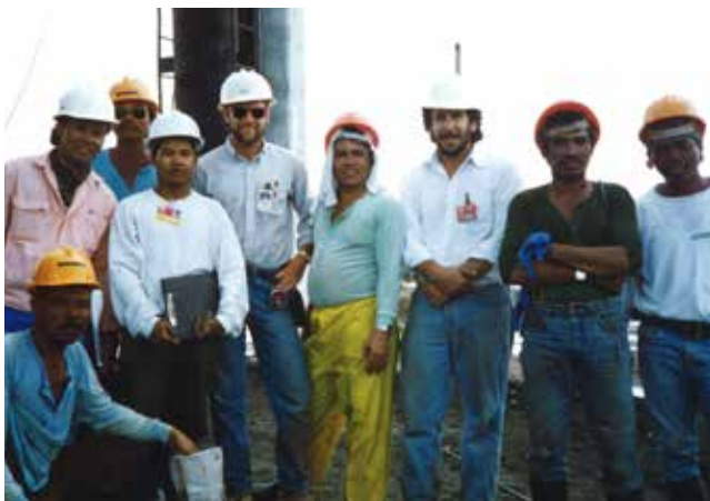
Driving driven precast concrete piles in Batangas, Philippines (1992).
