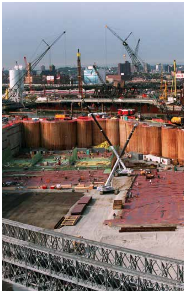
Cellular cofferdam for Boston's "Big Dig" project that experienced excessive lateral deformations.
