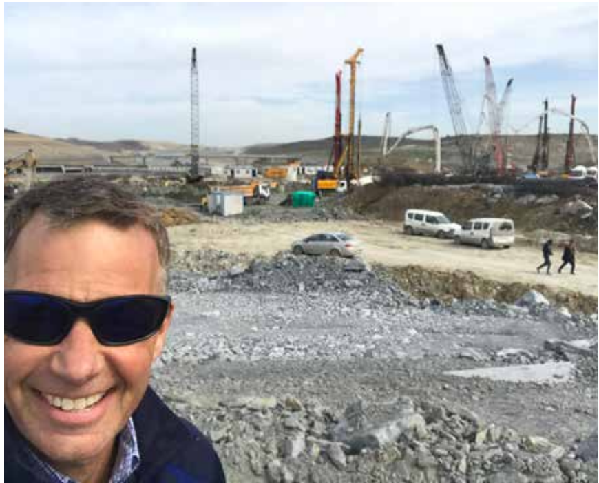
Geopier Impact Pier® jobsite visit for the new Istanbul International Airport project in Istanbul, Turkey (2018).
