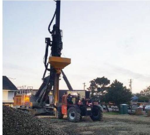
Due to the shallow groundwater table and potential caving soils, two displacement systems were used for this project. The Geopier Armorpack® system was utilized to penetrate through the loose sands and organic soils and bear on the medium dense to dense silty sand to support the footings and the Geopier Impact® system was used on grid pattern below the building footprint and a confining row around the building to mitigate liquefaction below the slab between footings.
