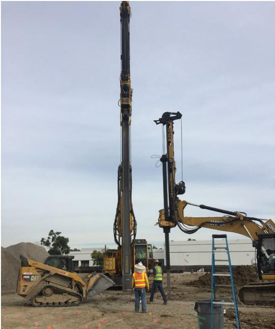
explorations. An innovative design solution combined the use of 24-inch X1® and Armorpack® elements to a depth of 35 feet to control static settlement and reduce the risk of construction delay caused by the caving soils. A total of 970 Geopier elements were installed to support the parking structure in 7 weeks.
