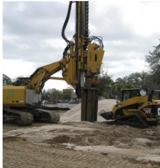
**Options:** One option proposed by the geotechnical engineer included supporting the structure on shallow spread footings and designing the structure to accommodate the total liquefaction and static settlement potential. Alternatively, ground improvement techniques including Geopier's Rammed Aggregate Pier® system to provide reinforcement, densification and drainage were considered. Geopier® also offered a solution using Rammed Compaction® soil densification using the Densipact® system.
