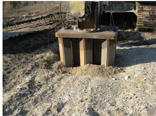
**Geopier Solution:** The Rammed Compaction® solution using the Geopier Densipact™ system was selected as the most cost-effective option for the project compared with the other traditional options. The upper topsoil was removed and replaced with compacted granular fill. 200 Rammed Compaction Points were installed to depths of 10 feet beneath the entire footprint of the tank and the ringwall foundation in three days to accomplish densification of the site.
