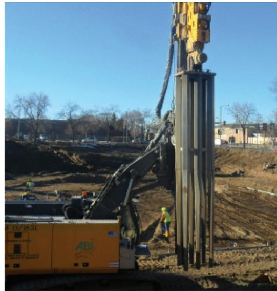
establish and adjust installation procedures to maximize improvement, especially for near surface soils where confinement was limited. The site was terraced at different working elevations, to improve performance and constructibility of the Rammed Compaction® Points (RCPs). Shallow supplemental RCP's were performed to enhance near surface improvement in elevator core. 504 Rammed Compaction® points were installed in eleven days, to complete the soil densification.
