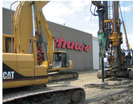
unsuitable fill and organic deposits. Specifically, 70 Geopier® elements provided support for spread footings bearing at an allowable design pressure of 4,500 psf and 71 RAP elements spaced at approximately 10 foot centers provided support for a four inch lightly reinforced concrete slab-on-grade. RAP locations were determined so as to avoid an existing 24 inch RCP storm drain that ran directly beneath the addition.
