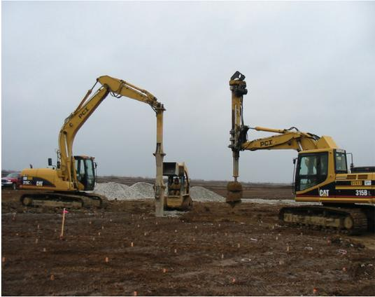
acceptable magnitude. Over 600 RAP elements were installed to depths of up to over 25 feet below grade to limit total settlements and control differential settlements beneath the tank floors and stem-wall foundations. Modulus testing for the project revealed less than 0.2 inch of deflection within the RAP reinforced zone at the maximum design stress.
