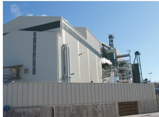
**Geopier Solution:** To limit settlement of the heavy structural loads supported over the thick deposits of compressible alluvial soils, the buildings and tanks were supported over Rammed Aggregate Pier® (RAP) elements in lieu of more costly conventional deep foundations. The GP3® solution incorporated 30-inch diameter RAP elements supporting up to 70 kips each. The foundations were designed as conventional spread footings utilizing an efficient allowable bearing pressure of 5,000 psf.
