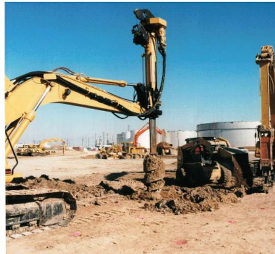
elements were installed around the perimeter of each tank within a zone extending 8 feet from the edge of the tank to the depth of 16 feet below existing grade. The RAP elements were constructed using Cement-Treated Aggregate (CTA). A factor of safety greater than 1.3 against edge instability was obtained and less than a 1/2 inch of settlement occurred after the Geopier system was installed.
