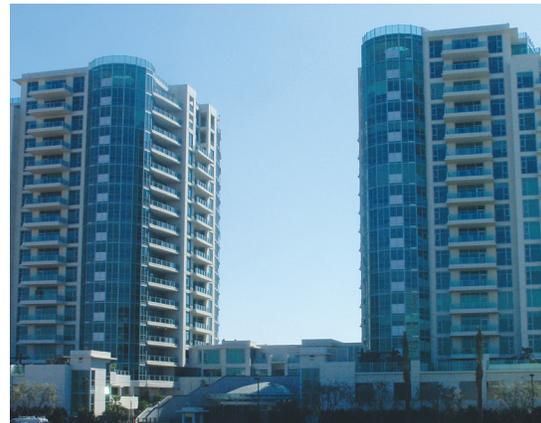
terminate in the underlying dense alluvial sands. A total of 1,850 Rammed Aggregate Pier® (RAP) elements were installed in 27 days. Two vibrating wire extensometers were installed beneath the mat of each tower to verify the compression of the RAP elements. To date, total recorded deflection is a maximum of ¼ inch within the Geopier zone.
