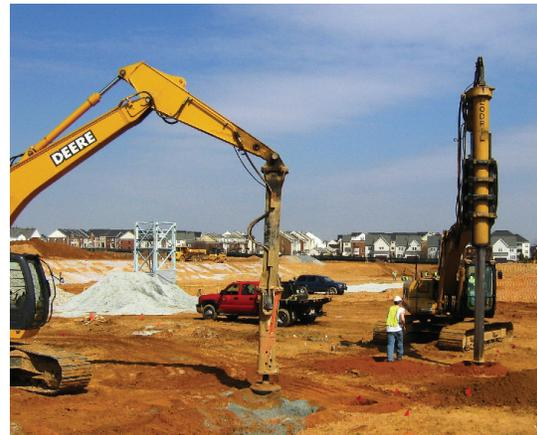
footings of 5 ksf in the poor soils to match the spread footings of 5 ksf in the natural soils so as to control differential settlement. More than 700 piers ranging in shaft length from 8 to 20 feet were installed. Two modulus tests revealed less than 0.36 inches of deflection at 100% of the design stress of 16,941 psf, reflecting the strength of the Geopier elements.
