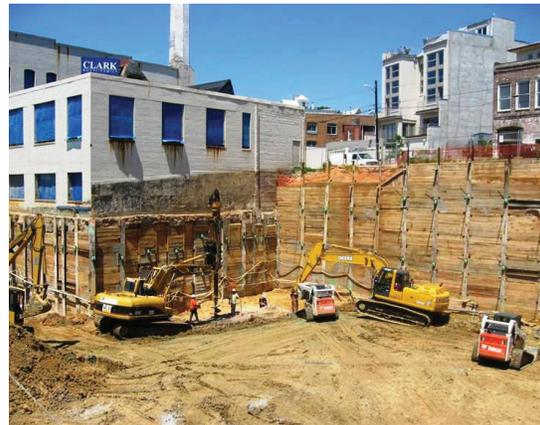
Aggregate Pier® (RAP) elements would be less costly than the 80-foot long drilled shafts that would have been required. Despite the challenges presented, the installation team was able to install a total of 375 RAP elements in 19 days. A modulus test taken during production revealed less than 0.49 inches of deflection at 100% of the design stress of 19,818 psf.
