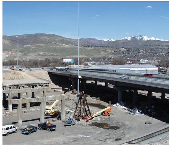
reaction frame. Also, piezometers were installed in the matrix soils between piers to monitor pore water pressures during the cyclic testing of the bridge bents. Prior to the GP3 installation, each testing site and both reactions frame sites were explored and evaluated by means of drilling borings, Borehole Shear tests, stepped land tests, and cone petrometer.
