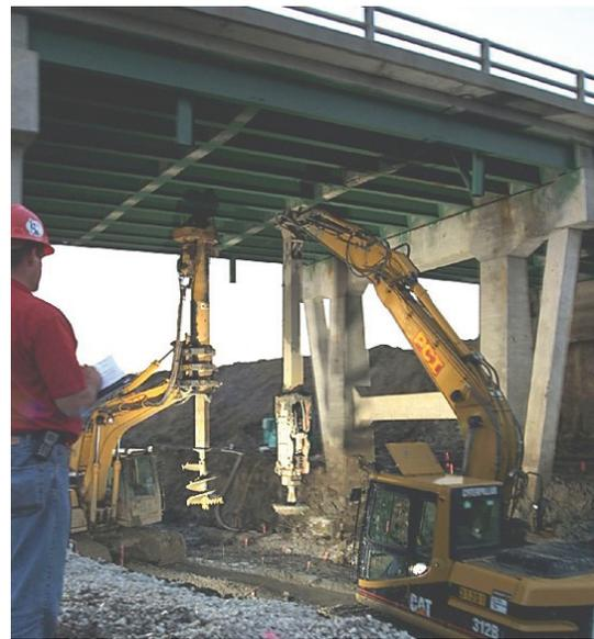
on-center. The Geopier design consisted of four different sections with elements of varying shaft lengths of 6.5, 14, 19, and 22 feet, corresponding to changes in fill height along the length of the culvert. Total and differential settlements were substantially reduced to within stringent project criteria.
