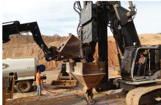
system and the upper 8 to 10 feet being constructed using the Geopier GP3® system. A total of 1380 RAPs were installed. The Geopier solution was verified with a modulus testing during production that confirmed a stiffness of 511 pci at a pier design stress of 14,400 psf.
