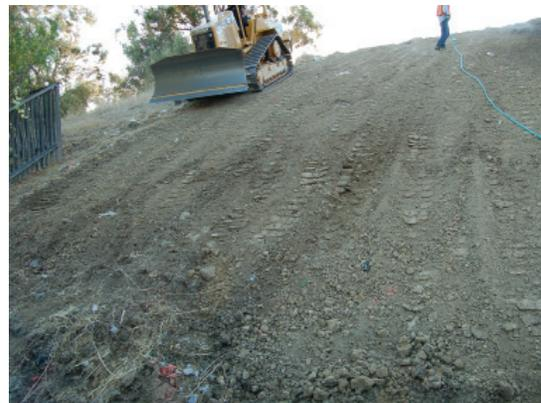
track rolled once again. Subsequently, jute erosion matting and wattles were placed over the slope for erosion protection.
