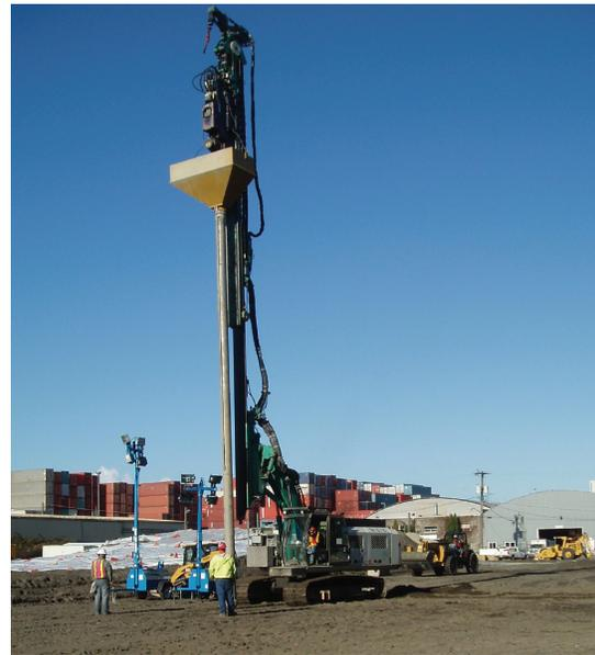
choosing the Impact system. Modulus test results showed about 0.21 inches of movement at top-of-pier stress level of 18,350 psf.
