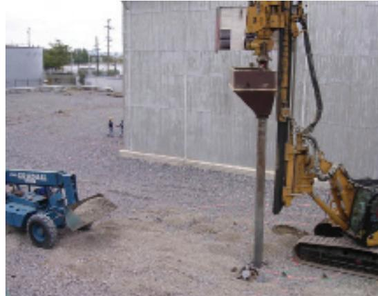
installed in 15 days to a depth of 18 feet to control total and differential settlement to 1" and 1/2" respectively, and to provide significantly greater liquefaction mitigation protection.
