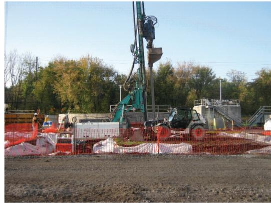
and equipment loads on top of the oxidation tank, grouted Impact® piers provided a more economical design. A total of 423, 20-inch diameter grouted Impact piers were installed to depths of 20 feet below the tank base.
