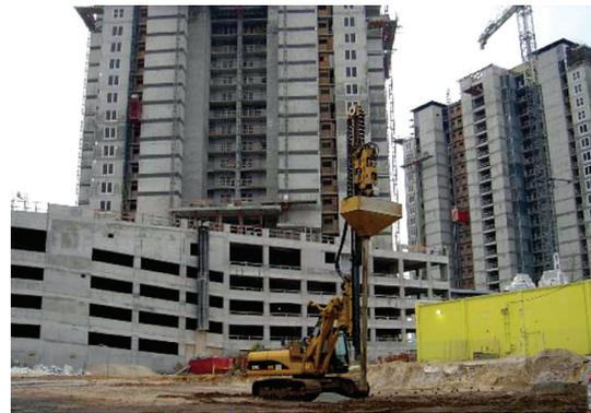
Unlike the augercast pile alternative, the RAP work could proceed while the building permit was being obtained. Installation progressed quickly even while grading and staking operations were still underway for some areas of the parking deck. The dry displacement Impact System proved very effective as the working pad had been cut 3.5 feet below finished floor elevation and was flooded by stormwater twice during the timeframe.
