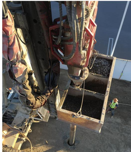
More than 1,300 Impact elements were installed to depths of 30 feet in only 29 days. An added benefit of the liquefaction mitigation program was reinforcing the soft clay layers and creating a 30-foot thick crust of reinforced soil to provide support for the mat foundation static loads.
