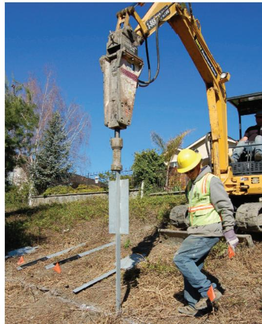
began while the slide was still moving. The excavator pushed the Plate Piles through the soft clay slide mass and then drove them the final four feet to a depth of 7.5 feet below the slope surface. The installation was completed in four days with minimal disruption to slope vegetation and auto traffic.
