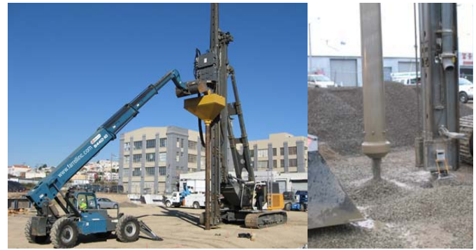
Fig. 2: Impact pier equipment with standard rammer head
