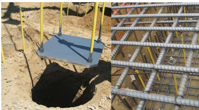
Fig. 1 RAP Uplift Bottom Assembly and Top Anchor
