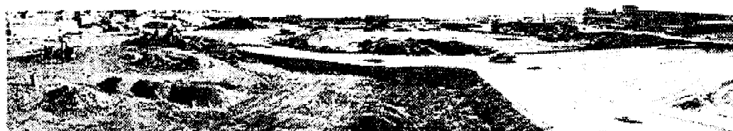
Figure 1. Rammed Aggregate Pier construction (left), preload (right)
