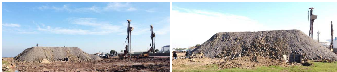
Figure 14. The test embankment field photos.
