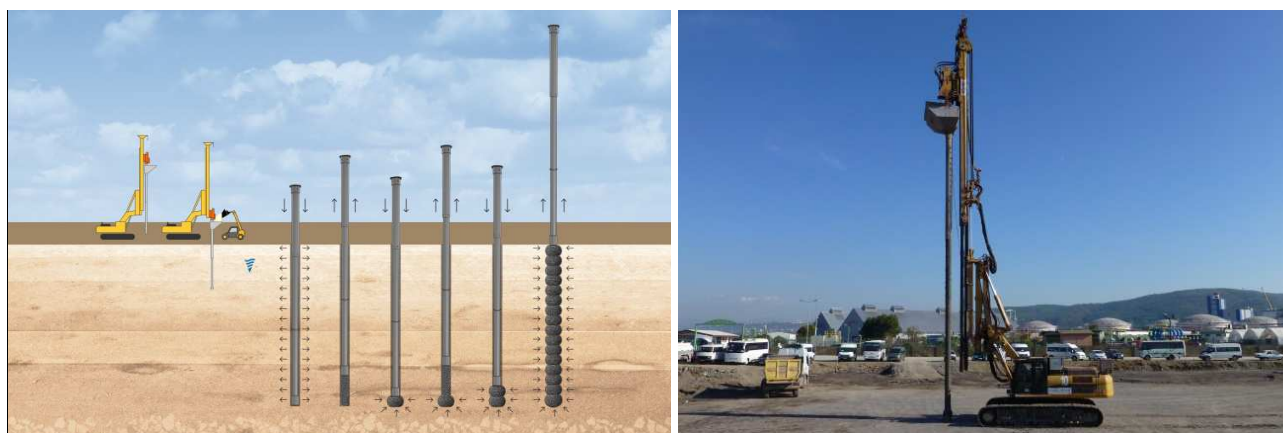
Figure 7. Construction methodology of RAP Impact elements and a view from the field construction.
