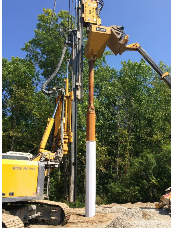
Figure 2. Confined aggregate pier construction.
