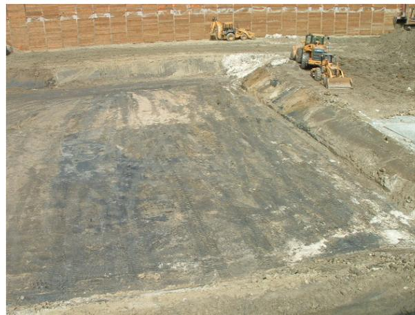
Figure 1. Excavation at base of west tower showing compressible clay layer
