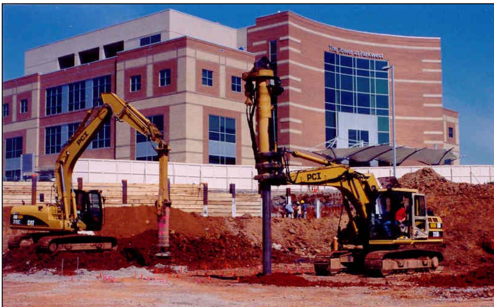
Figure 6. Geopier Construction at Project Site
