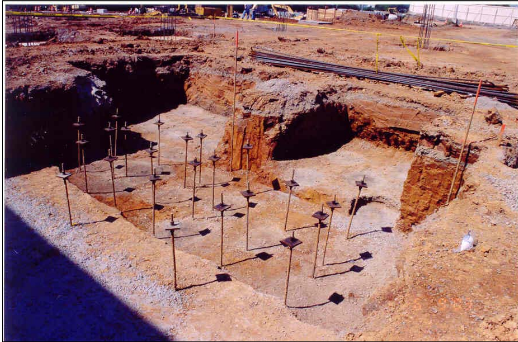
Figure 5. Uplift Anchor Rods in Subgrade
