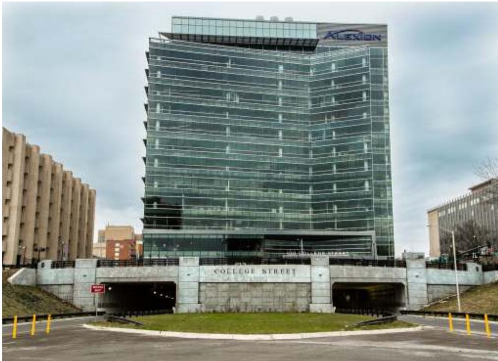
Figure 2: Photo of completed structure, illustrating Route 34 below the building, central core loading and “outrigger footings”
