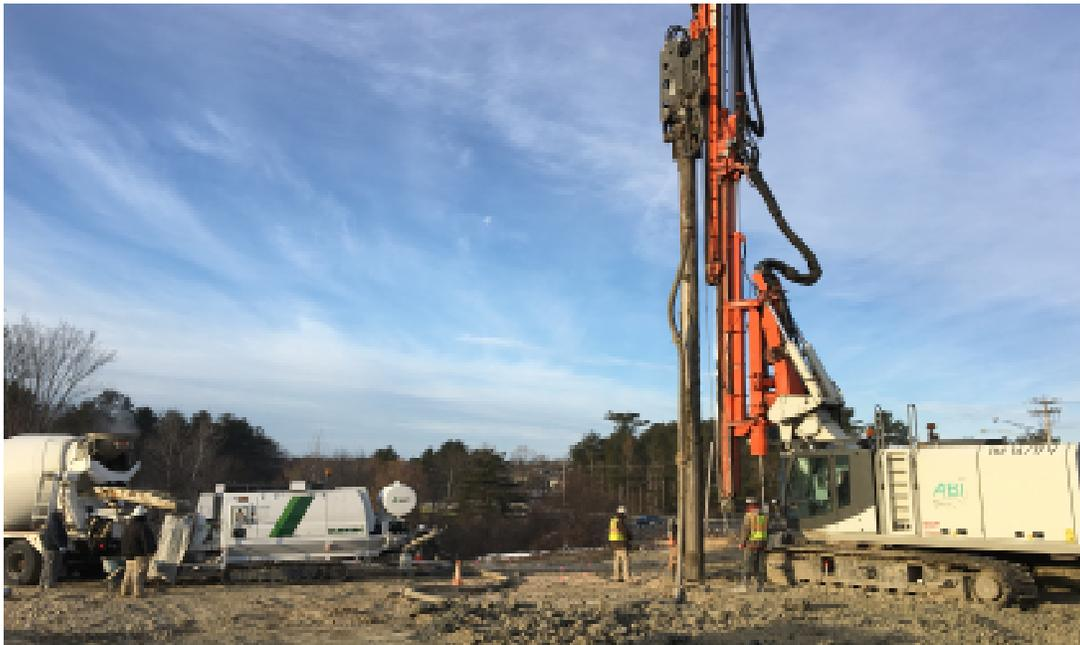
Figure 7: GCC Construction Equipment, including ABI mast rig, concrete pump, concrete truck
