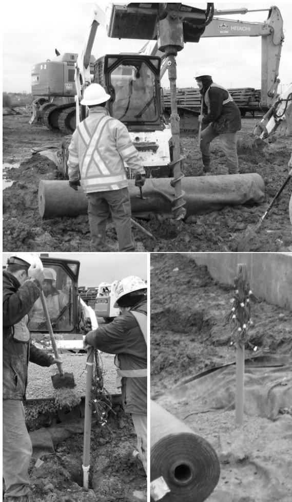
Figure 4. Temperature sensor installation
