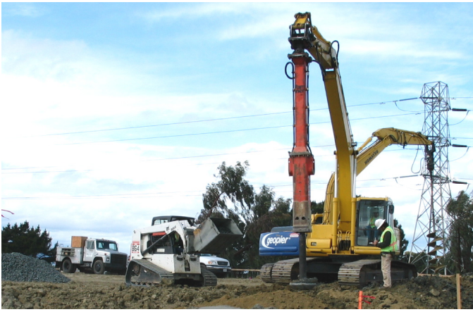
Fig.7. Typical RAP Installation Equipment
