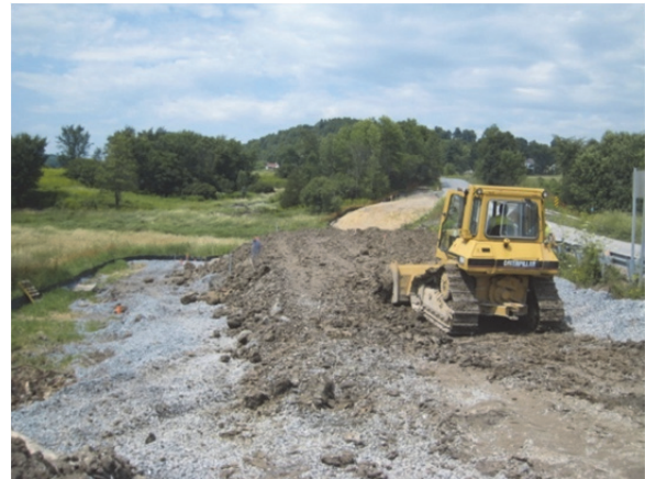
Figure 7 – The Clay Fill was only compacted during placement with a Dozer.
