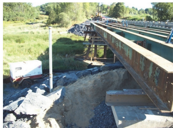
Figure 8 – Abutment Bearing at Top of Embankment.
