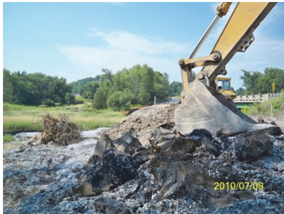
Figure 5 – “Controlled” Placement of Clay Fill
