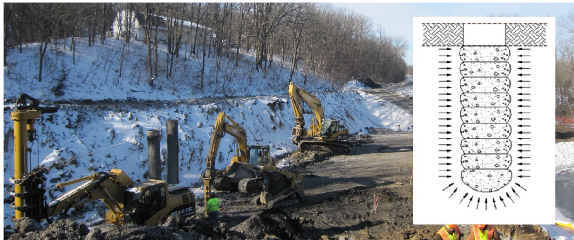
Figure 5. Several Geopier installation rigs were mobilized to perform the construction. The increase of lateral stress adjacent to installed RAP elements is shown schematically in the inset, at right.
