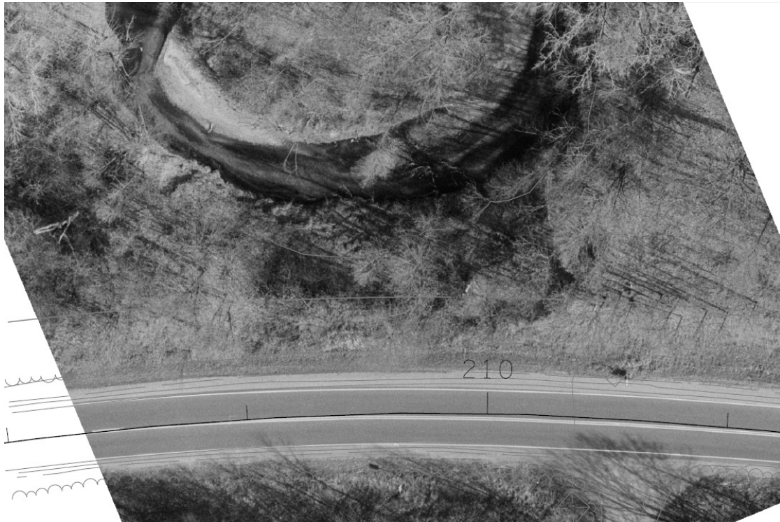
Figure 2. The north side of the MN 67 highway embankment is adjacent to an outer stream bend of Hazel Creek. Progressive channel erosion on the outside bank of the stream appears to be a contributing factor in the movement observed on inclinometer T-100 [lower left, approximate station 208+75] and the long-term small-scale ongoing pavement distress seen from 1998 to 2010. Significant new movement and roadway distress occurred after a large rain and flood event in September of 2010.
