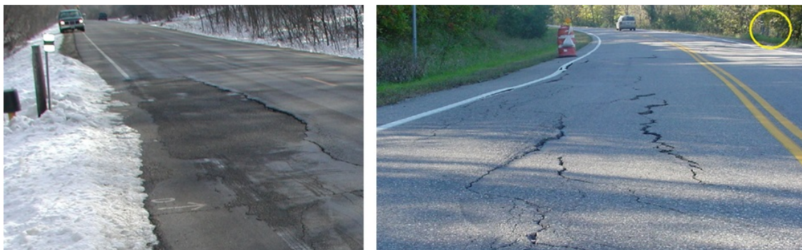
Figure 1. The roadway asphalt was patched sometime prior to January of 2007 (left). The 2010 distress, (right), propagated across the entire MN 67 roadway. The T-100 inclinometer installation [at left in the left photo] can be seen in the upper right of the right photo [yellow circle] taken from the other direction.
