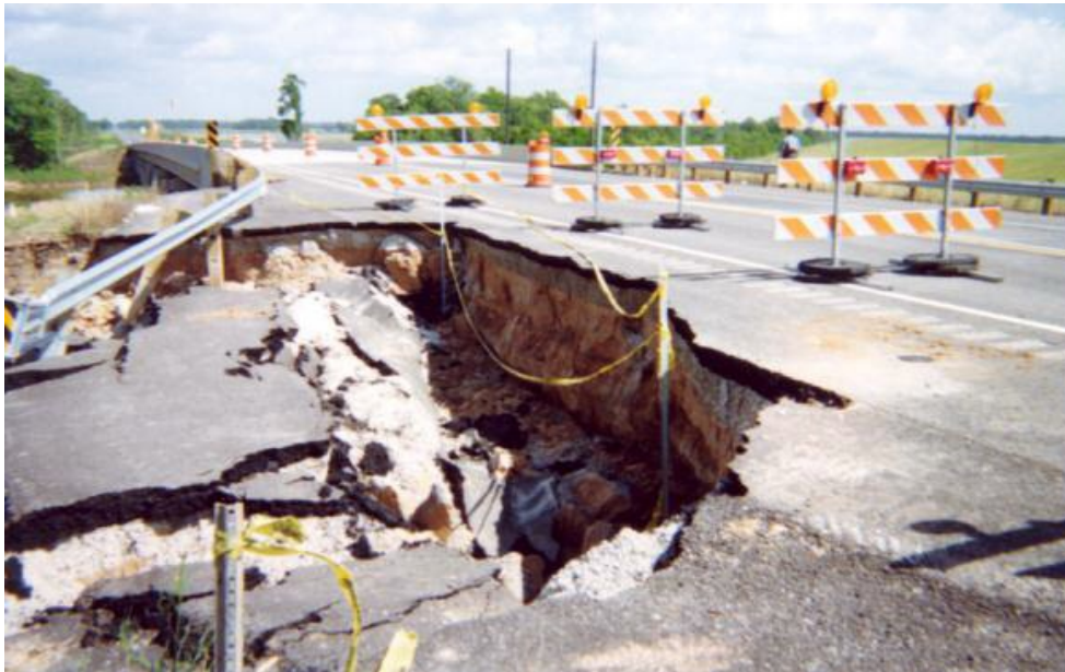
Figure 2- Slope Failure at US-71, Krotz Springs, LA
