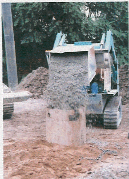
Figure 3. Dumping a pre-measured amount of aggregate that when compacted will comprise a single lift in the pier.
