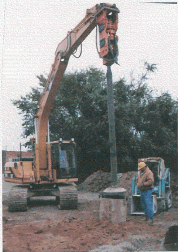
Figure 4. Special beveled ram being lowered through the temporary casing to compact the next layer of the aggregate pier.
