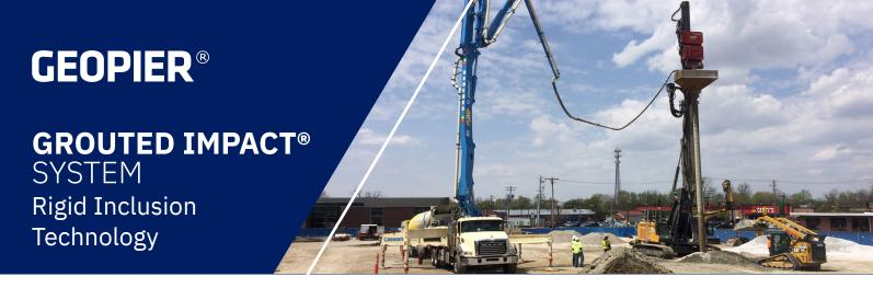
The Geopier Grouted Impact® system uses our traditional Impact pier with grout added to the open-graded aggregate during installation. Grout is introduced to the system within the mandrel and mixed in place to create a high-strength grout-aggregate mix. The end result is a very stiff, cemented pier element that provides confinement in weak soils and excellent settlement control for heavily-loaded structures.
