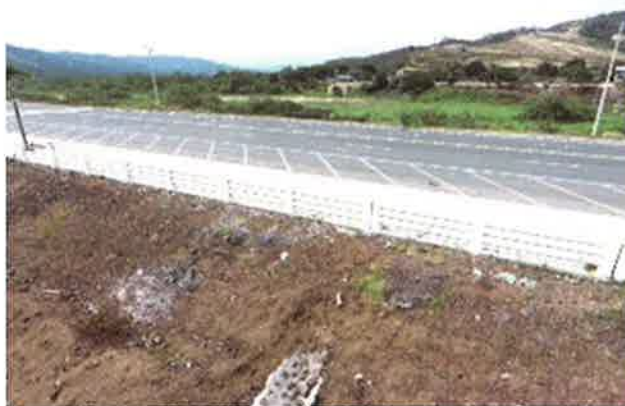
Figure 5. Briceño River Bridge Approach Embankment supported on RAPs after the earthquake.
