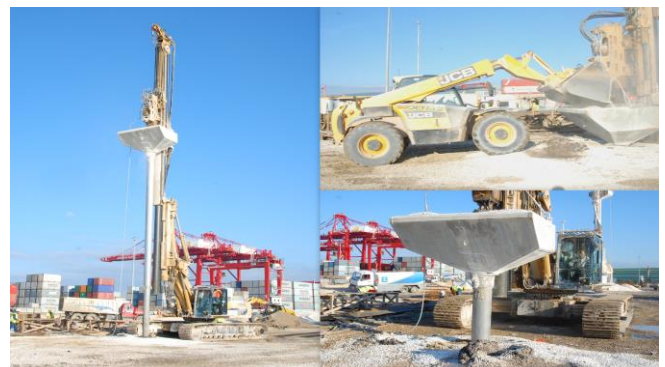
Figure 1. Construction of Impact ® Piers
