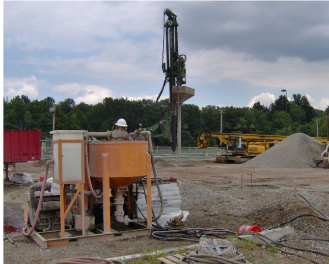
Figure 5. Grouted aggregate pier construction
