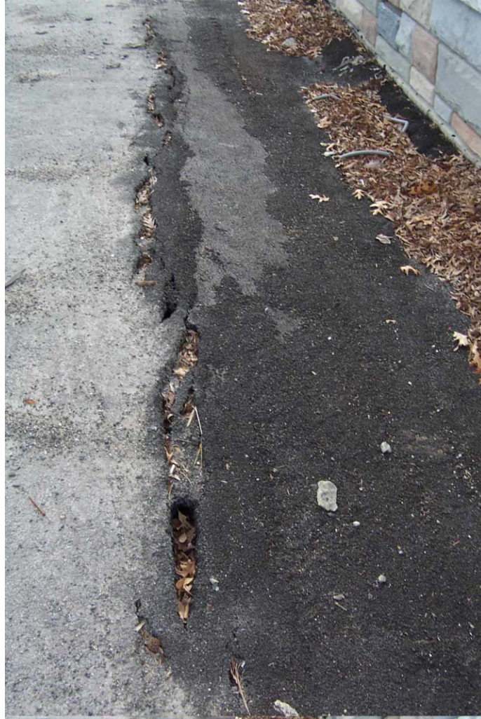
FIGURE 4. Photograph showing distress in the roadway behind concrete barrier wall
