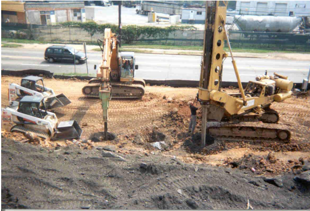
FIGURE 12. Rammed aggregate pier construction
