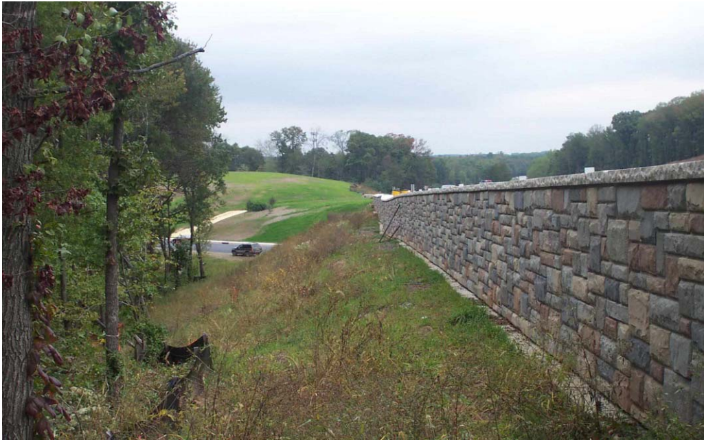
FIGURE 3. Photograph of failed slope area
