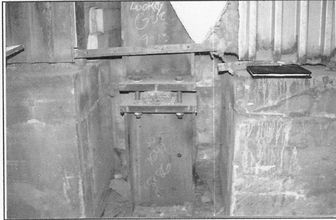
Figure 1: Structural repairs required as a result of foundation movements
