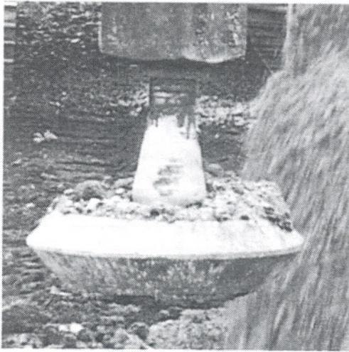
**Fig. 1.** Rammer used for layer compaction of Rammed Aggregate Piers
