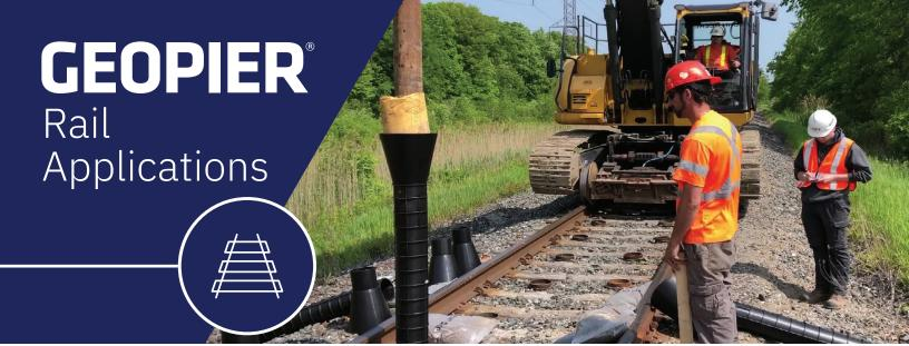
FOR TRACK MAINTENANCE APPLICATIONS, THE GEOPIER GEOSPIKE<sup>SM</sup> AND SRT® SYSTEMS ARE RAPIDLY INSTALLED, LOW-COST METHOD FOR STABILIZING RAILROAD SUBGRADES.
