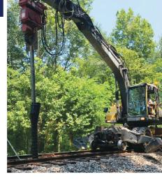
**NORFOLK SOUTHERN** DEMOPOLIS, AL Approximately, 120 GeoSpike<sup>SM</sup> elements were installed in the 200' section in a day and a half resulting in 0.14" deflection at 150% design load.
