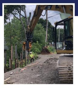
STREET SLIDE REPAIR Plate piles were installed in one day to repair a shallow slide adjacent to a roadway in Norwalk, OH without any interruptions to traffic.
