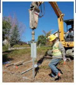
**PROGRESS SLIDE** Winter rains in San Ramon, CA resulted in a 200 ft x 50 ft shallow slide. SRT was used to stabilize the slide mass in under 4 days for less than \$60,000.
