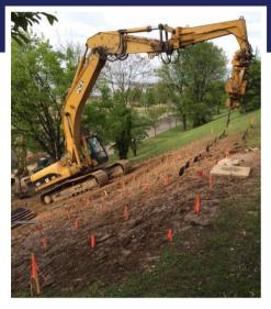
MUDSLIDE REPAIR 250 Plate Piles were installed in Memphis, TN to stabilize a slope after a heavy rainstorm dropped 8 inches of water.
