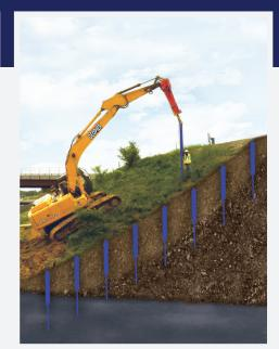
**SLOPE REINFORCEMENT** The Geopier SRT<sup>®</sup> system is used to stabilize slope failures or reinforce marginally stable slopes
