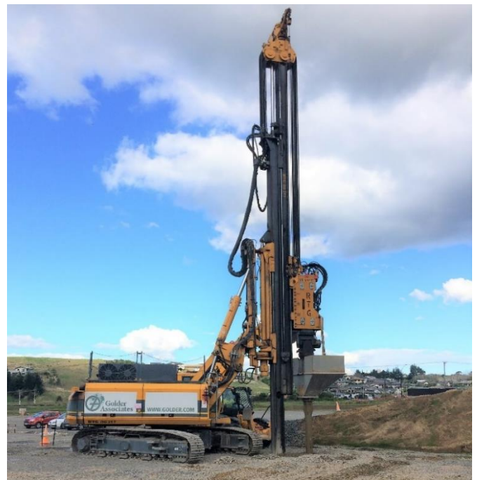
Figure 5: RAP installation rig at Tauranga Crossing.
