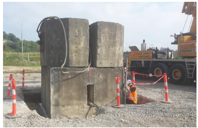
Figure 9: Footing load test
